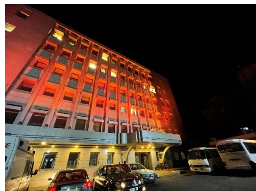
The façade of the University Pediatric Hospital in Damascus was illuminated in celebration of World Patient Safety Day 2021
