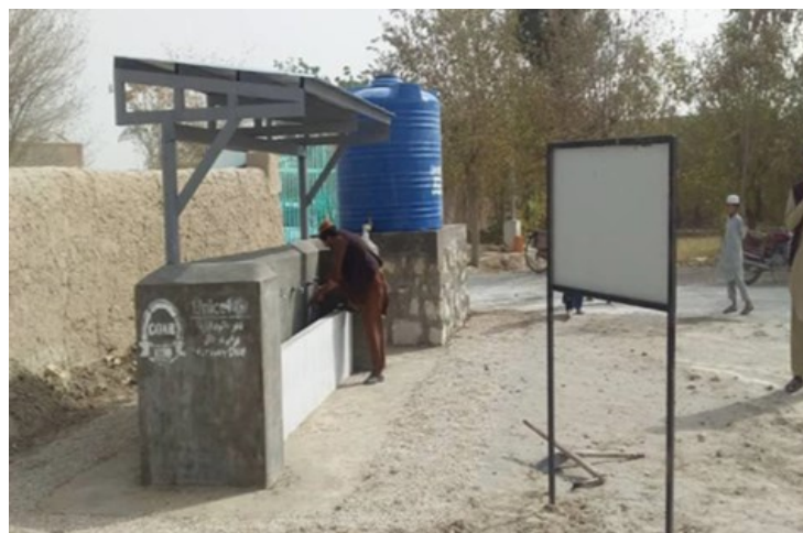
Figure 6. Handwashing facility at Manjigak clinic, Jawzjan, Afghanistan, Sep 2022
